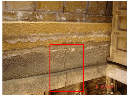
The damaged stone has been restored to reconstruct the gateway
