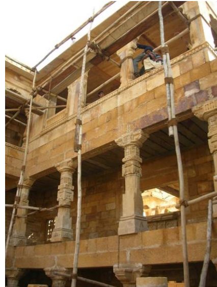
Columns and Arches after restoration
