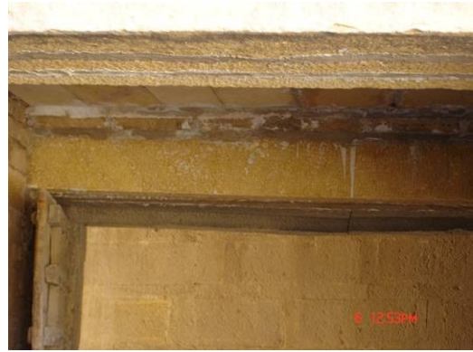
Load has been transferred by placing a new girder over the existing lintel
