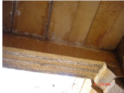
The stone slabs have been restored and neatly joined to form the gateway
