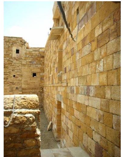
Out of Plumb Payaga wall restored with proper verticality.
