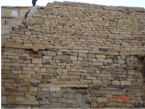
Wall over Gateway has been reconstructed after complete dismantling
