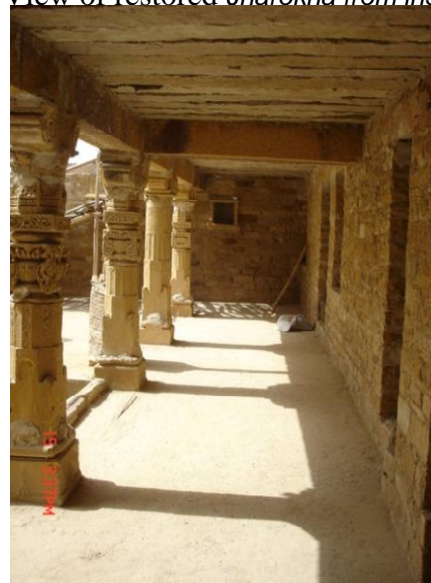
Stone slabs in Roof – Second floor
