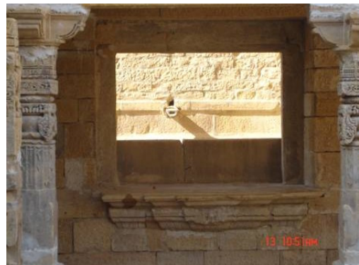
View of restored Jharokha from inside
