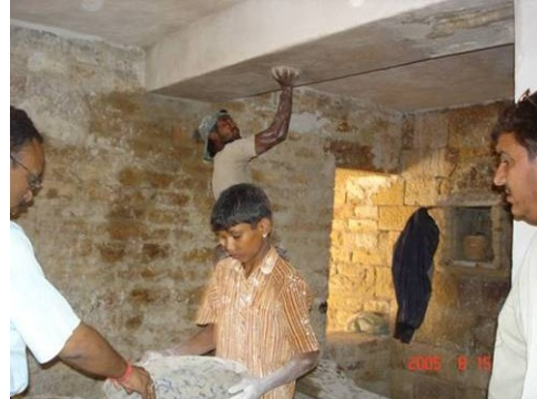
Inspection of quality of Lime paste by the Architect
