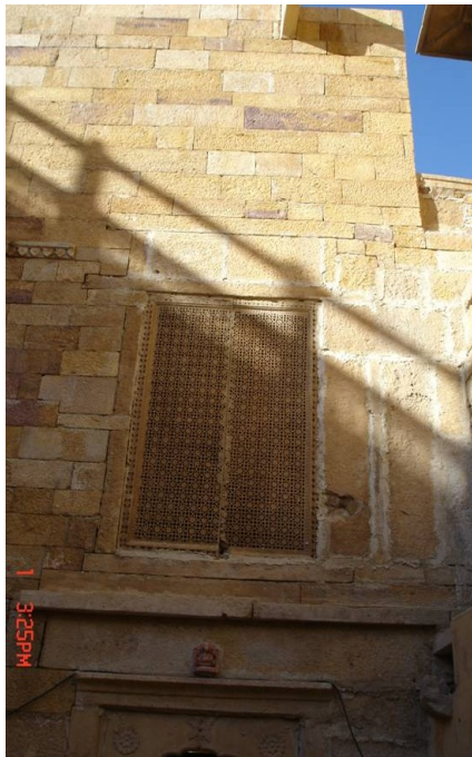
Wall above gateway to staircase
